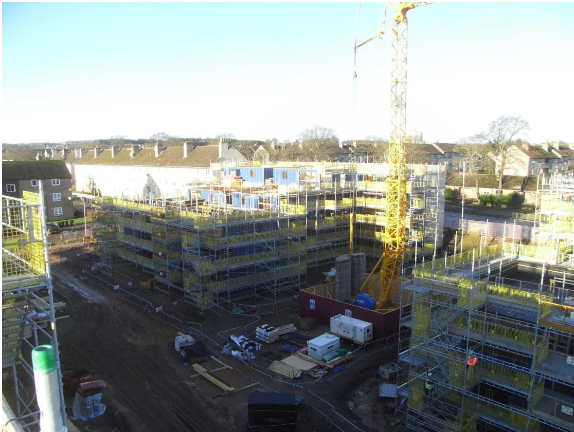
Block 1 – Timber kit erected to top floors; roof to commence (02.12.2020)
