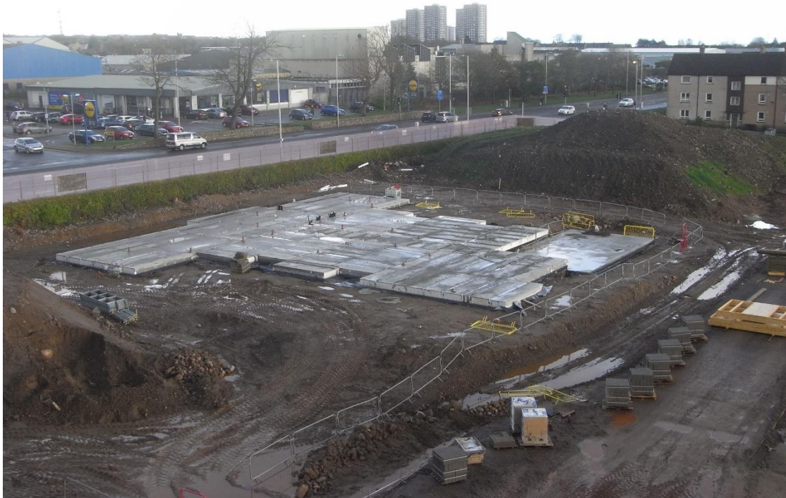
Block 3 – Foundations complete (12.11.2020)
