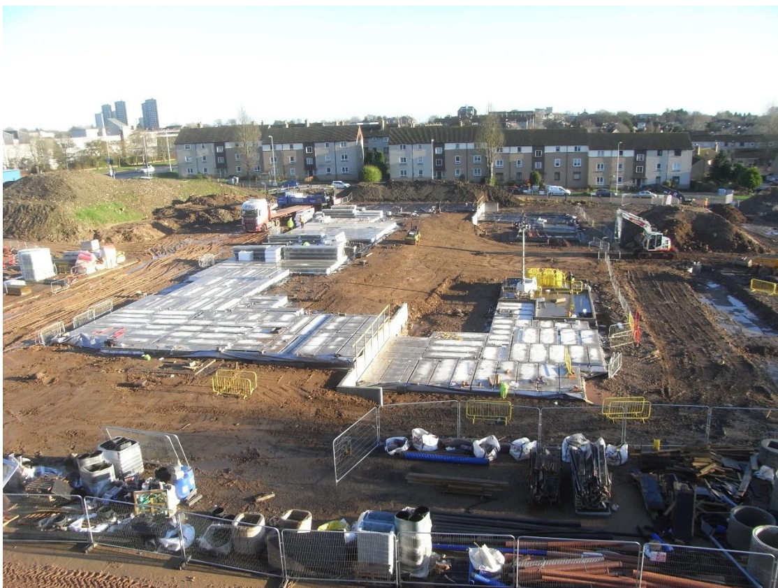
Block 6 – Foundations in Progress (02.12.2020)
