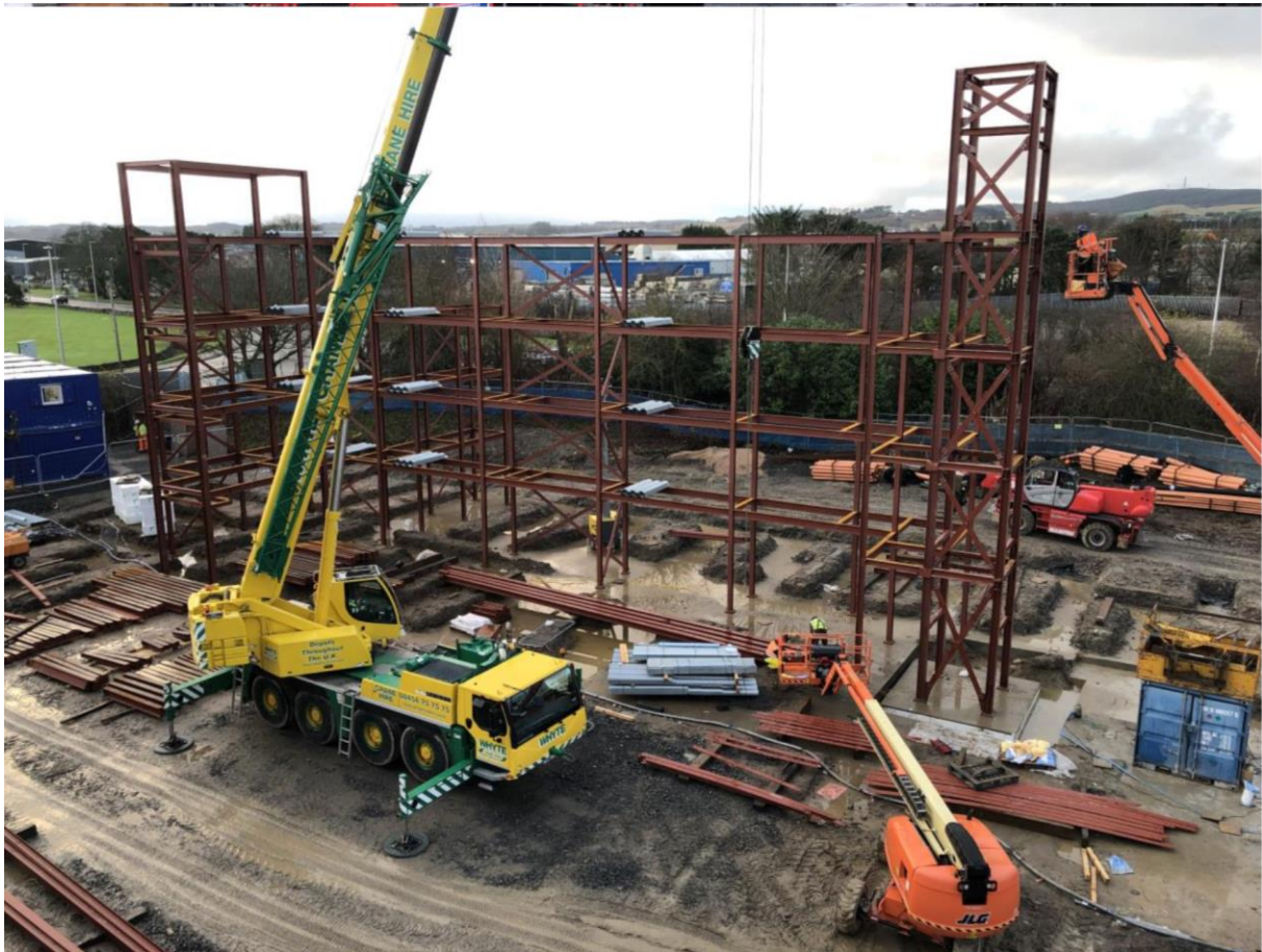
Block 1 – Superstructure/ Steel Frame progressing (15.12.2020)
